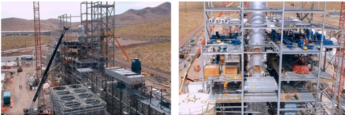
Construction photos of Sierra Biofuels plant. (Source: Abengoa/LinkedIn)
